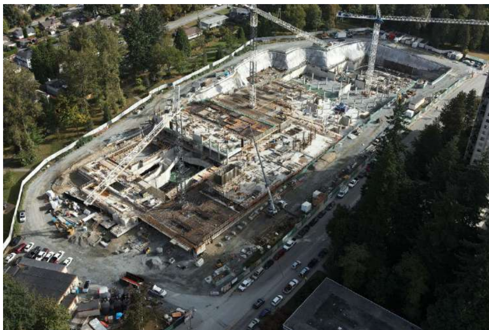
New Cameron construction
