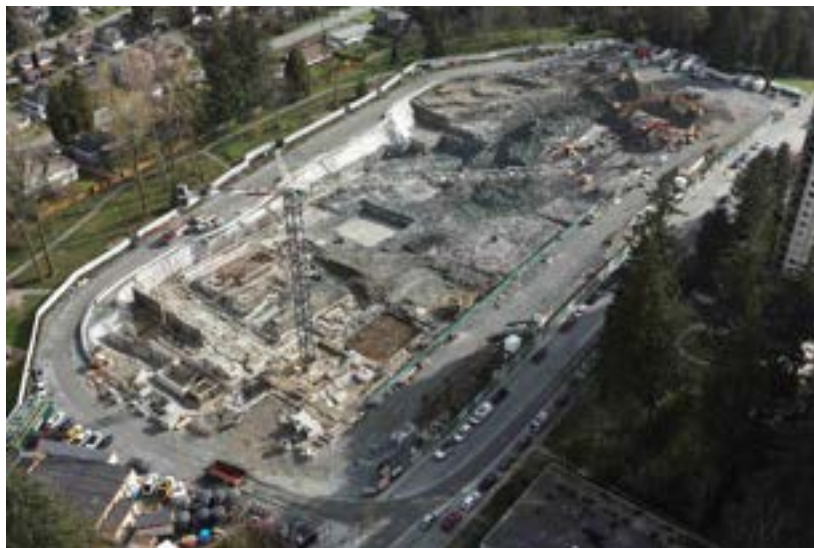
New Cameron construction site
